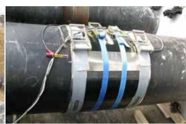
The connection of the pipes is the weak link in a district heating system, which is why post-insulation of the highest quality is necessary. Our electric fusion sockets are setting new standards in socket technology. They ensure force-locking, waterproof and firmly bonded post-insulation due to the homogeneous welding to the pre-insulated steel pipe.
