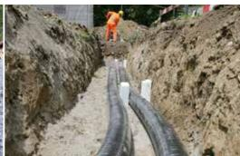
Delivery lengths up to 810 metres on one coil and highly flexible pipes simplify routing. Short construction times and small trenches minimise construction costs.
